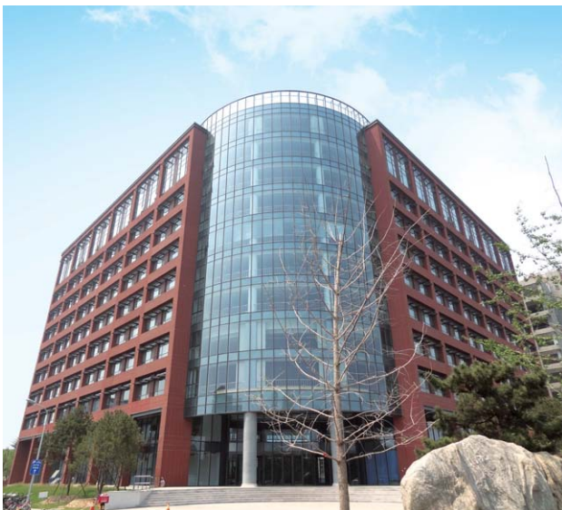
Tsinghua-ROHM Electronic Engineering Hall
