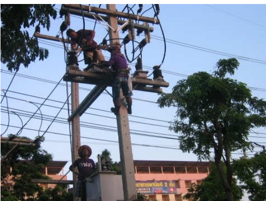
The power company works to reconnect power.
