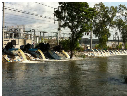
Water is pumped out of the industrial park.
