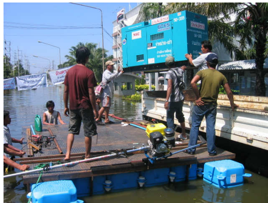
Workers bring in a temporary generator.
