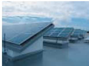
ROHM Apollo solar energy generation facility Annual power generation capacity of 24,000 kwh
