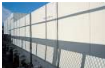
Ice thermal storage air-conditioning system
