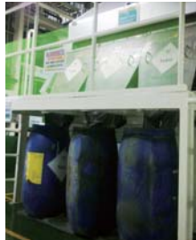
Drum Dryer at REPI
